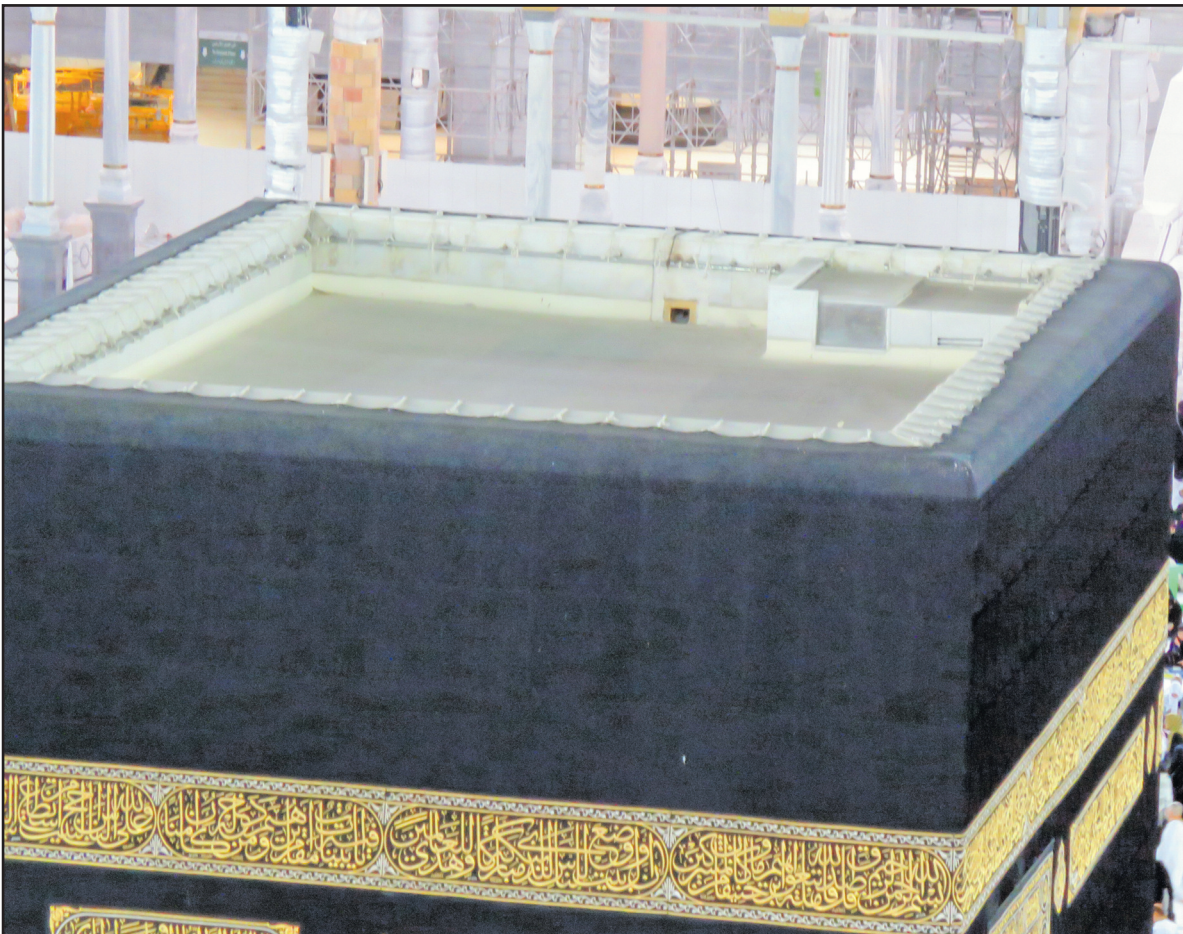
The box-shaped roof of the Kaabah leads to water accumulation, hence the need for the meezab to allow the water to flow away.
